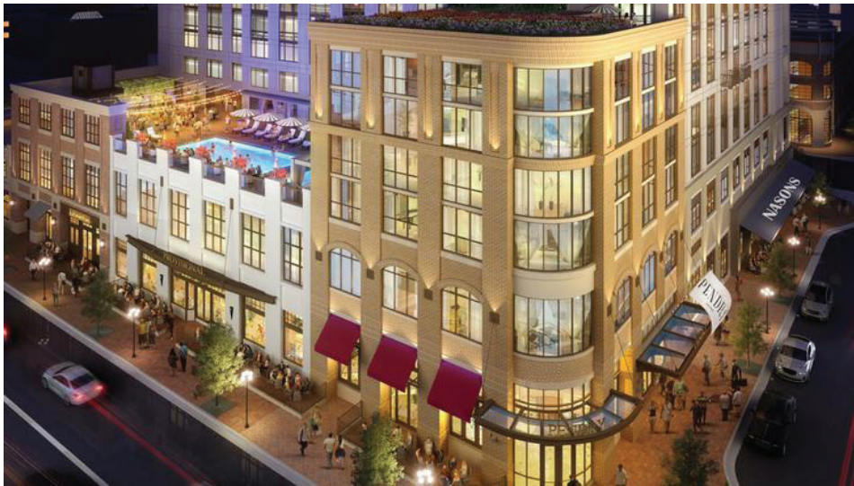
Depicted in this rendering, the Pendry Hotel is due to open next week in downtown San Diego. It is one of eight hotels that were under construction last year in the county.
